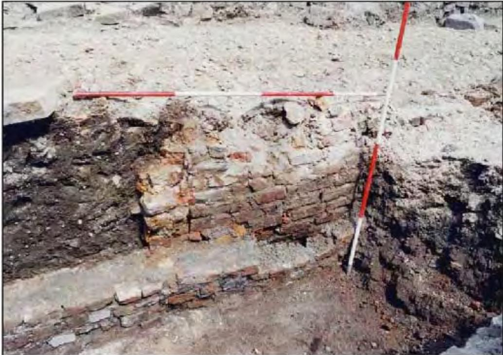
Plate 19 Detail of F19 wall with F70 garden soil exposed behind (left)
